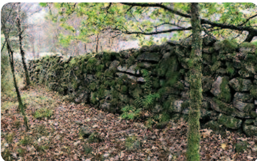
The parish stone wall in Eivindvik.
