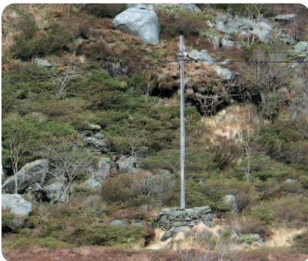
Telephone pole on elaborately designed foundations. Photo: Anne-Karin Mjse
