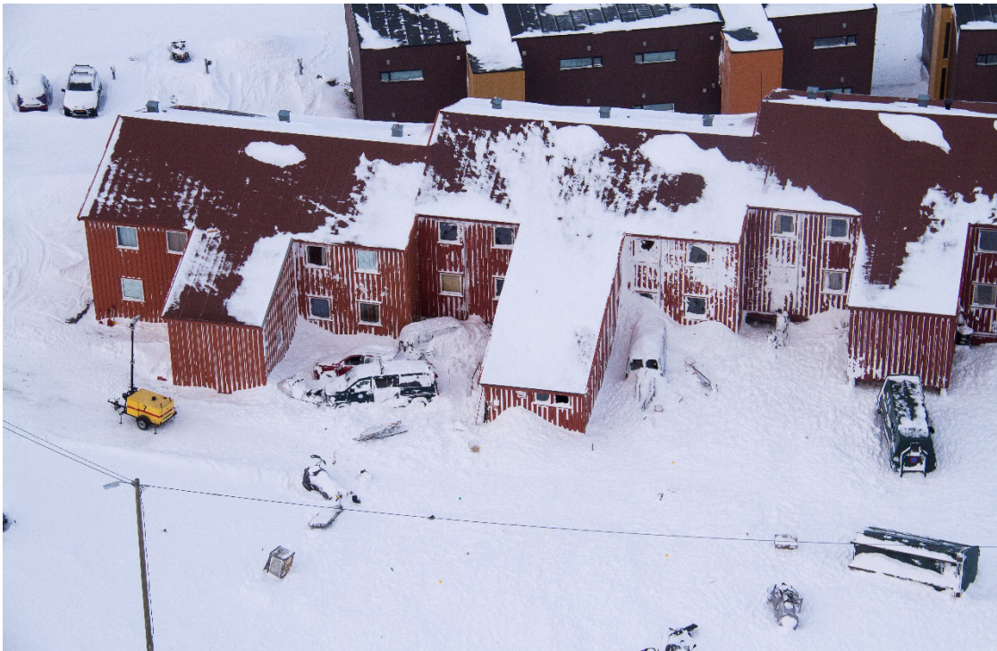
Photo 6.3.4: House 228/7-11 after the 2017 avalanche. Photo: Sysselmannen.
