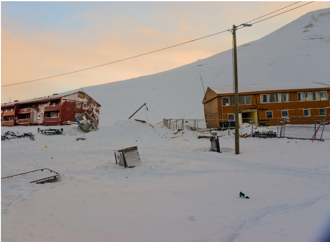
Photo 6.3.2: Road 228 after 2017 avalanche. Photo: Christian Jaedicke.
