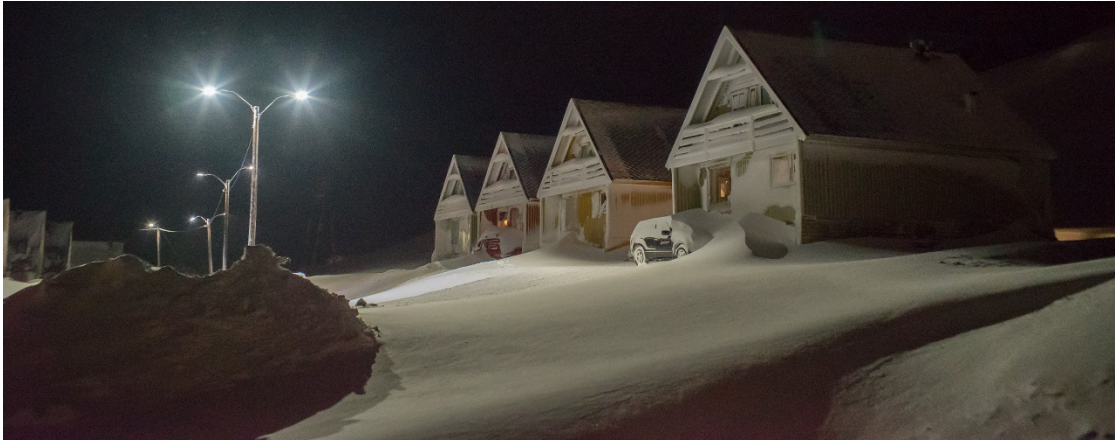
Photo 5.3.3. The upper row with 4 houses and street light below just before the avalanche. The two closest poles were completely destroyed by the avalanche. Photo: Tommy Markussen.
