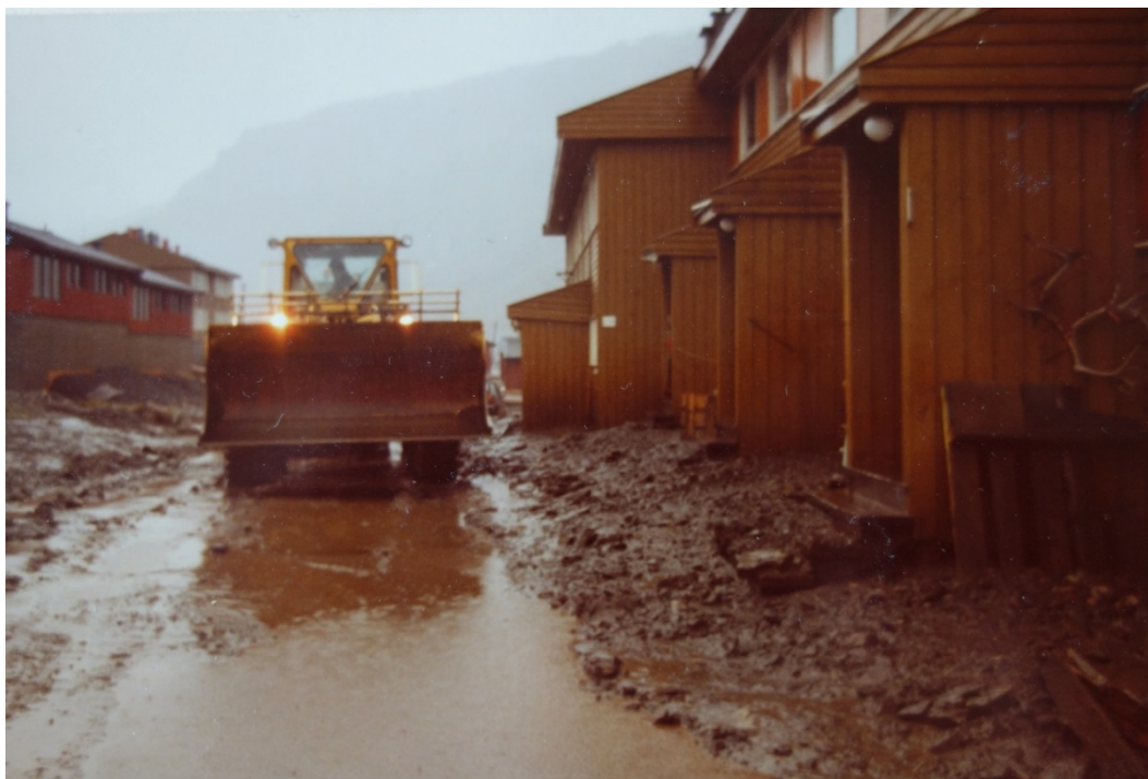
Photo 2.1: Debris flow in August 1981 causing damage on buildings in road 228 (6-16). Photo: Turid Telebond.
