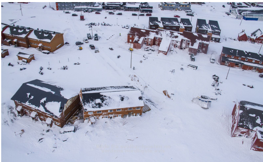
Photo 6.2.2: Aerial photo of 2017 avalanche. Photo: Sysselmannen.
