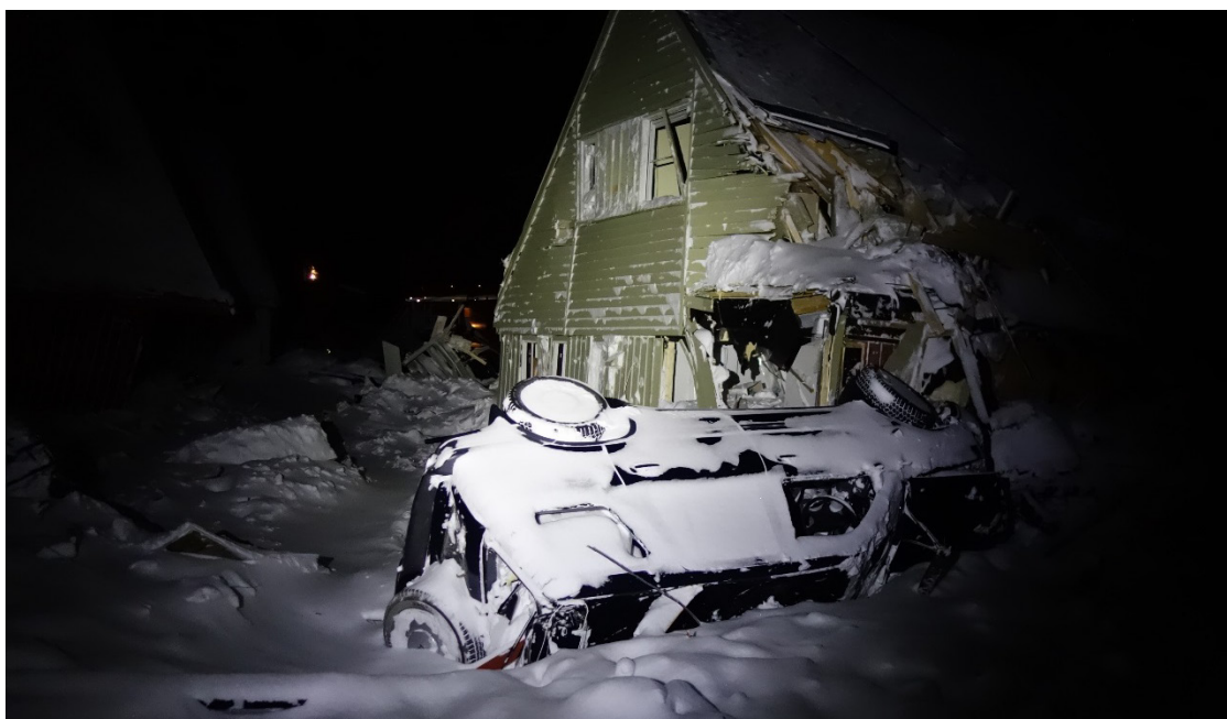
Photo 5.3.1: Upper row house 230/30 moved 80 m by the avalanche. Photo: Kjetil Brattlien.
